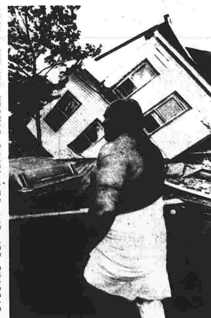
James Silvestri, who was taking a shower when his East Boston home suddenly collapsed Thursday, wears a towel as he walks past the ruins of his house. Four other occupants of the house were injured. The cause of the collapse is under investigation. (UPI photo)
