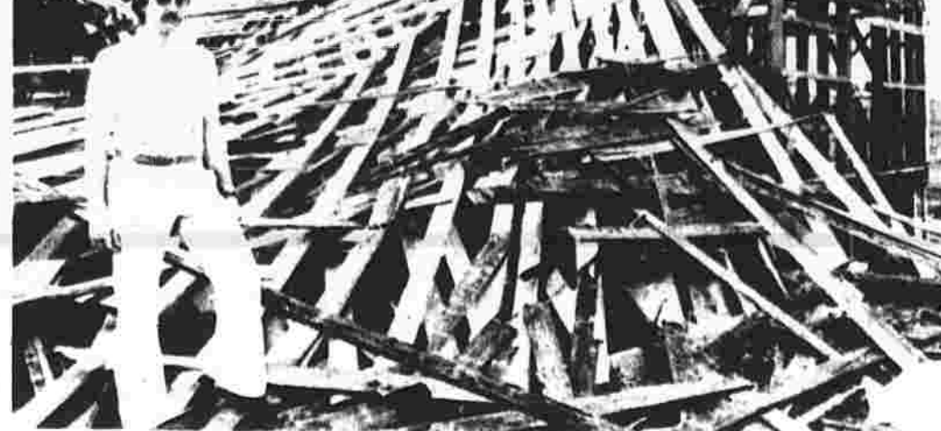
Steve Green, executive director of Living History Farms, surveys damage done Wednesday by high winds to a pioneer church being built in the site where Pope John II held an outdoor mass in 1978. The sanctuary portion of the Church of the Land was collapsed by 60-mph winds, part of a storm system that swept the state. (UPI photo)
